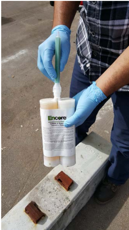
Using threads, screw on mixing chamber
